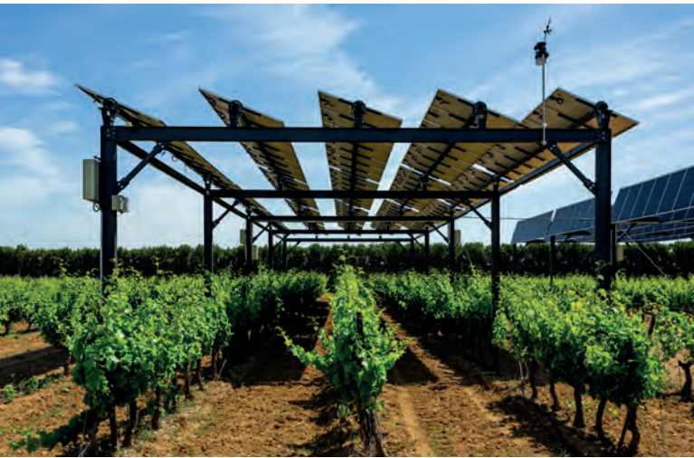
Fig. 31: Agrivoltaic system with solar tracking PV modules in France © Sun'Agri
