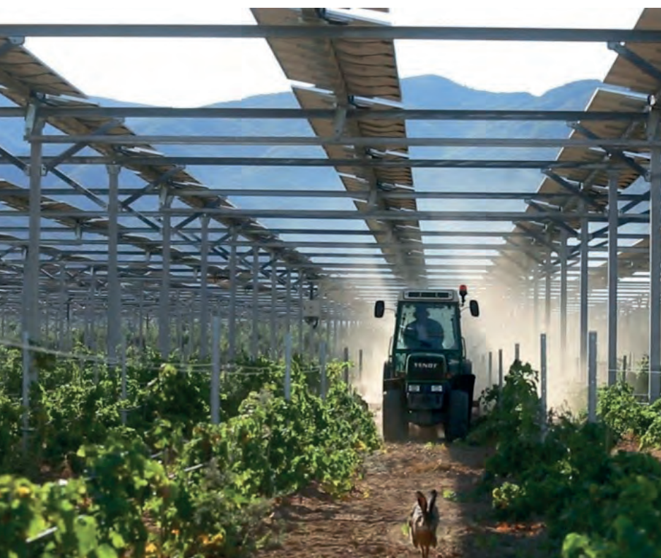
Fig. 49: Tilted, overhead system with continuous rows of modules © Sun'Agri
