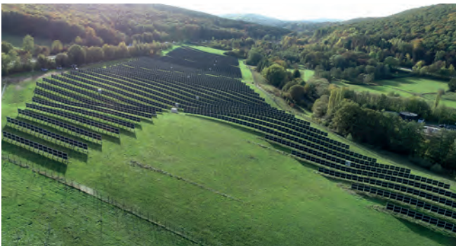
Fig. 57: Eppelborn-Dirmingen solar farm with 2 MW p with vertical solar fences by Next2Sun © Next2Sun GmbH
