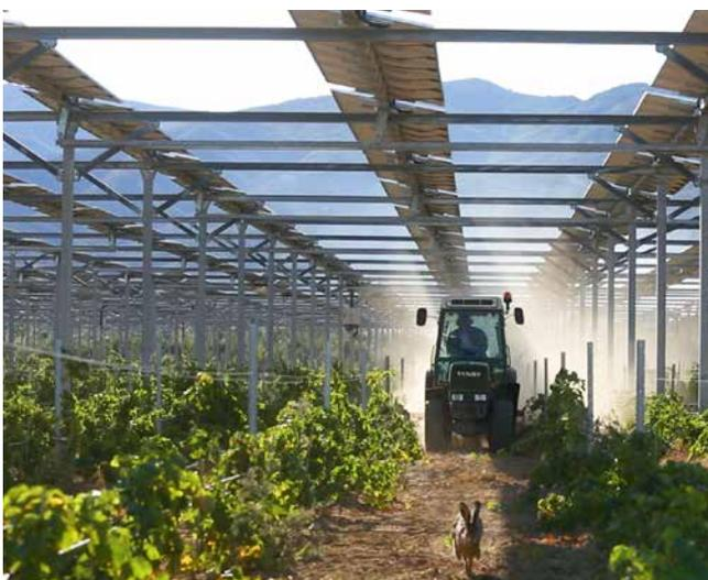
Figure 40: System with high mounting structure and continuous rows of PV modules. © Sun’Agri
