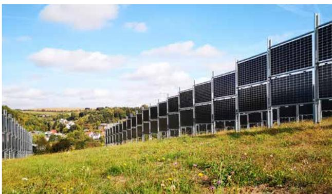
Figure 35: Bifacial modules installed vertically, Donaueschingen.
