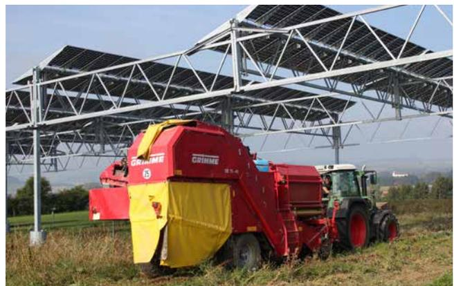
Figure 34: System with high mounting structure, permitting cultivation underneath the modules with the potato harvester.
