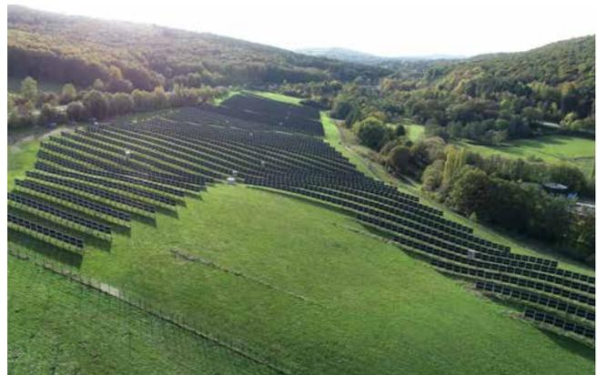
Figure 47: 2 MW<sub>p</sub> Solarpark Eppelborn-Dirmingen with vertical PV modules by Next2Sun. © Next2Sun GmbH
