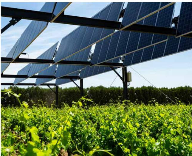
Figure 41: Single-axis tracking system of a demonstration agrivoltaic system in France. © Sun'Agri
