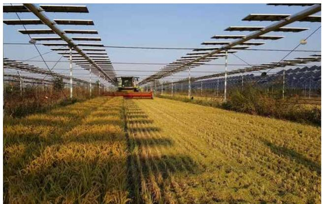
Figure 39: System with high mounting structure and narrow PV modules. © REM Tec
