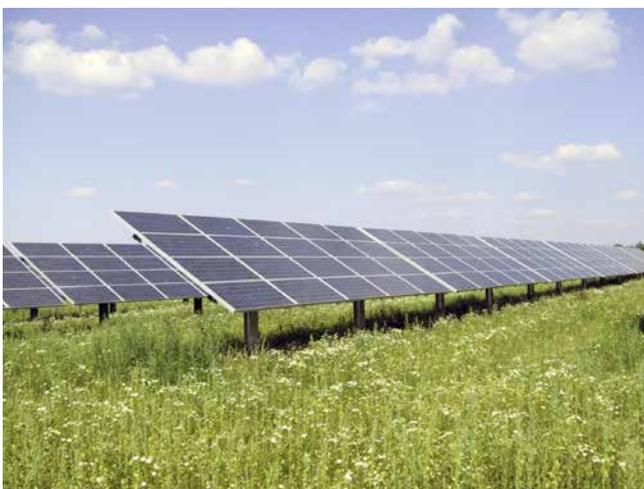
Figure 7: Ground-mounted PV system. © Fraunhofer ISE
