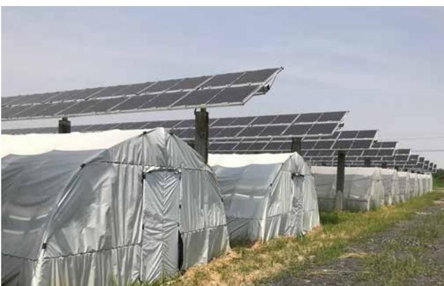
Figure 36: PV modules over a foil tunnel.
