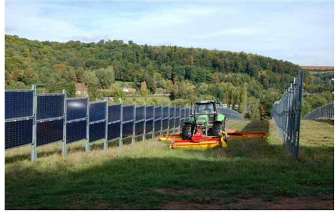
Figure 27: Vertically oriented bifacial modules in the Eppelborn-Dirmingen solar park, Saarland, with 2 MW<sub>p</sub> capacity, constructed by Next2Sun GmbH. © Next2Sun GmbH
