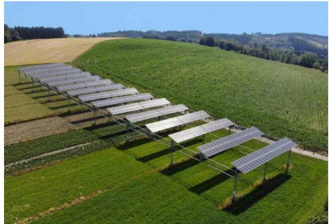
Figure 46: Agrivoltaic system in Heggelbach with 194 kW<sub>p</sub> capacity. © BayWa r.e.
