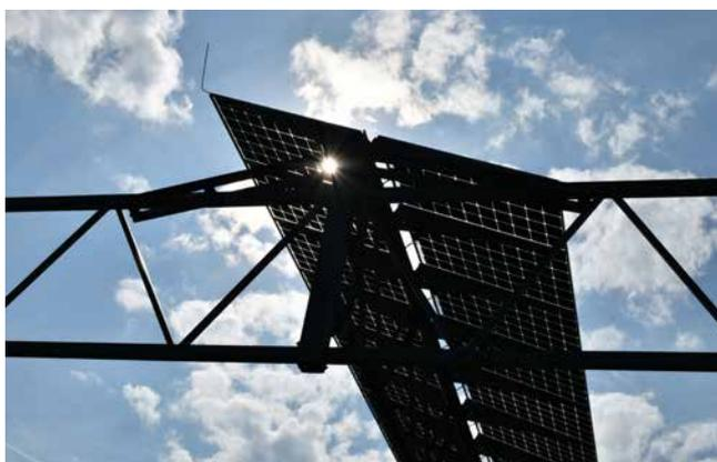
Figure 14: Module rows with bifacial modules at the agrivoltaic system in Heggelbach. ©Fraunhofer ISE
