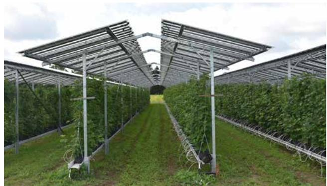
Figure 33: PV modules with spatially segmented solar cells and protective function in the Netherlands. © BayWa r.e.
